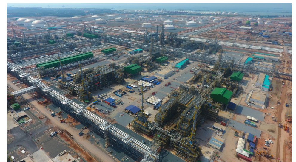
Pengerang Integrated Complex, Johor, Malaysia
